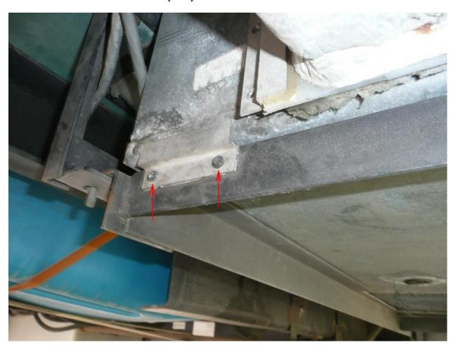
7. Check the seal of the aluminum tape about 1.5 foot up the duct work. In my case the whole 90 deg elbow fell to the ground because the alum tape adhesive had dried out. I had to cut about 3 in of alum tape off and re-taped with "Venture Tape". Venture Tape is very expensive (\$35/roll), but it is designed to hold duct joints permanently in very hot/cold attics.
