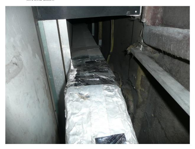
8. Use a bungee cord to hold duct back about an inch so the foam seal is not torn off.
