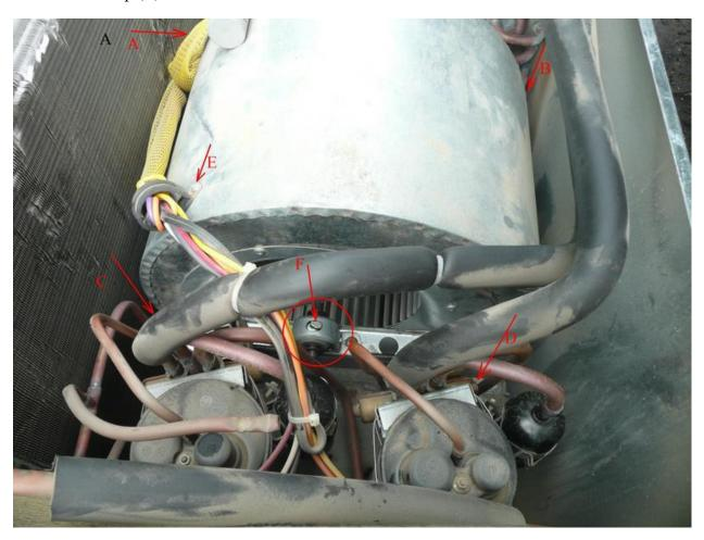
15. Lubrication point of the brass bearing of the indoor blower assy.
