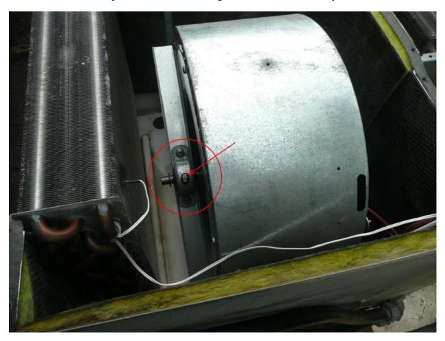
16. To remove the blower assy, pull the cable bundle up and out over the coils on the left. Have a helper hold the coil out at the top about 1 in (A) and push against the rubber covered copper line to provide a little more clearance so as to NOT touch and damage the coil fins on the left. Once pulled up to clear the 4 studs, the blower assy can be rotated and lifted out. It is a tight fit so take your time and don't bang up the delicate alum fins.
