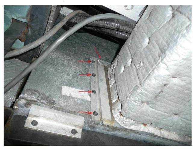
5. Remove the 5 screws on the right side of duct. A short 6" screw driver is useful on the top 3 screws. Have a helper hold the power cables back out of the way to aid access to screws.
