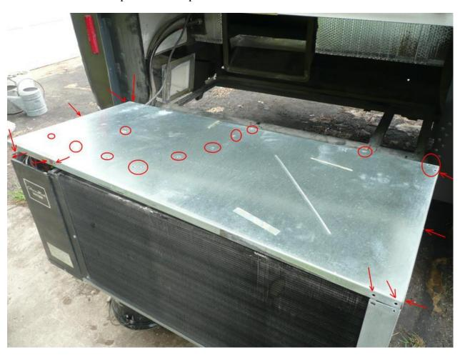
24. Before re-assy, tape up the ends of the two pieces of stryrofoam to temporarily hold while the unit is re-inserted.
