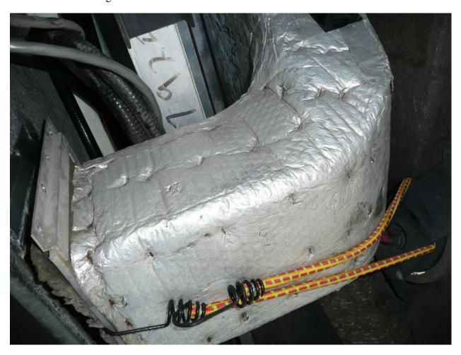
9. To push the unit out, I got on the green carpet under the unit. On my back I used my feet to slide the unit out about 1-2 inches, and then slightly raise the unit and slide out about 6 to 8 inches. There are several screws sticking out the bottom about 1/4 in and these hit and drag over the bottom supporting brace. Once the unit is out this far, then pull the power and control cables out so they will not get caught on the duct work.
