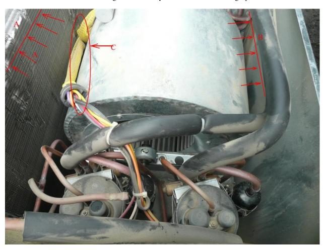
17. Remove the three power wires at this connector. The connector is labeled Common (White), Hi (Black), and Lo (Red).
