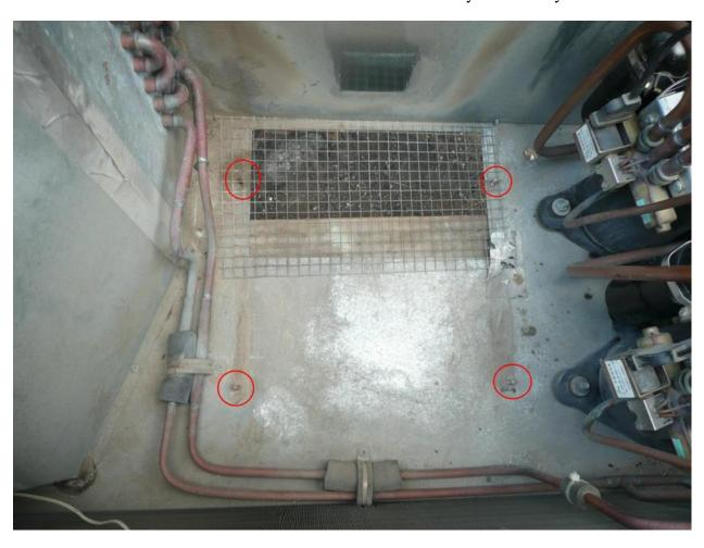
21. Use reverse procedure to re-install the blower assy. Use a little sticky butyl rubber on the nut to hold in the 7/16 socket to get the nuts started.
