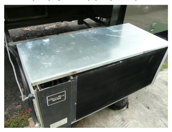
12. Take off the top cover by removing the approx 28 screws.
