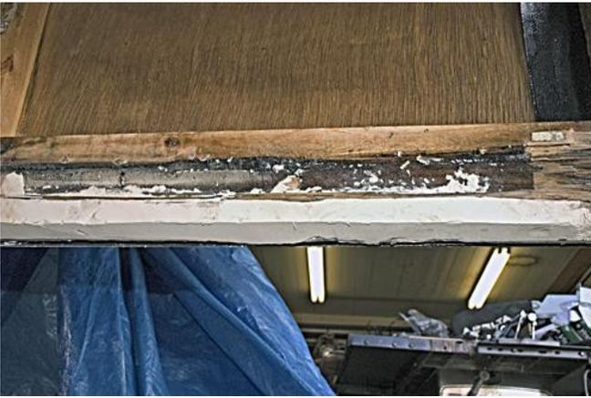
Yesterday it was too cold to work outside but it warmed up today. I sanded the framing member at the bottom of the exterior wall of the slide-out, squaring it so the plywood will lay smooth and the trim will fit properly at the bottom of the wall. I then installed the plywood gluing and stapling the luan. I had to cut out around the metal splicing plates. Turned out to be a good fit.
