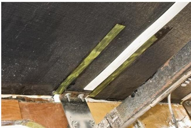
We finished her up today with the possible exception of the stripped cuts in the weather barrier. They might need another coat of resin, but they look pretty good. We put the trim on the bottom of the exterior wall of the slide and connected the electrical. Overall, the job looks pretty good.
